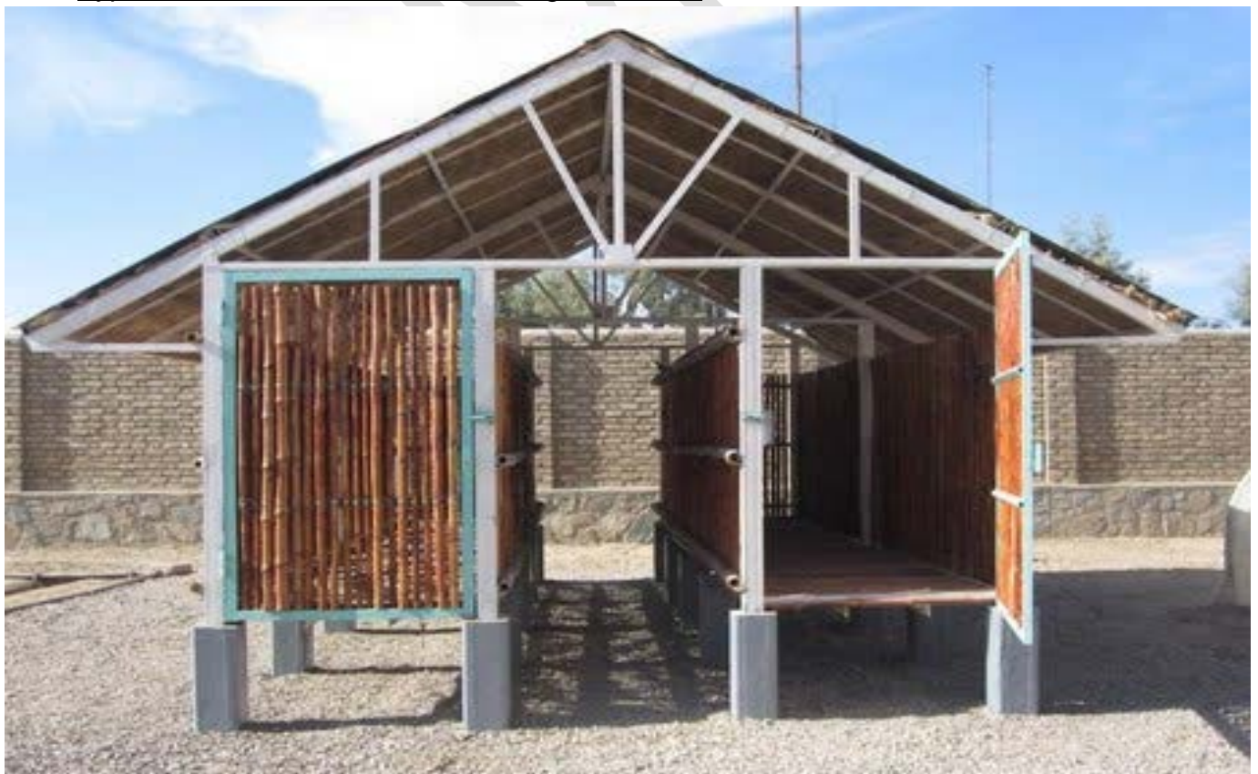
Typical Model of 50 MT Onion Storage Godown:
